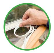
**Draught Stopping** Replacing or installing draft stopping to any leaky doors and windows can stop cold air coming in, and warm air going out.
