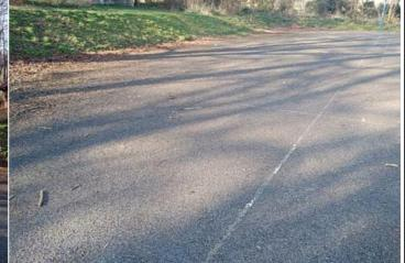
**Finding:** The surface is crumbing in areas creating slippery **Action:** Sweep and clear all loose debris and monitor conditions
