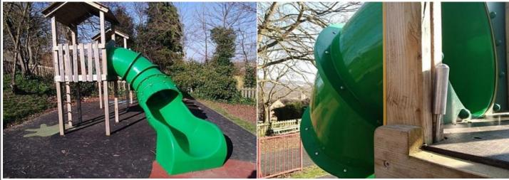
**Finding:** There is/are finger entrapment/s in the framework **Action:** Monitor - No remedial work recommended the item fails to meet the requirements of BS EN 1176 Part 1
