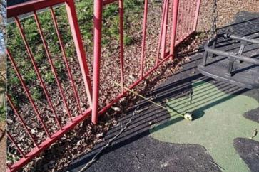
**Finding:** The seats are too close to the frame as defined in BS EN 1176 Part 2; this is a low risk failure and no remedial
