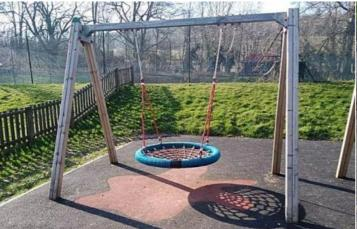
**Finding:** The seat clearance from finished surface level to the underside of the seat is too low when measured in its most onerous position and does not meet the requirements of BS EN 1176 Part 2
