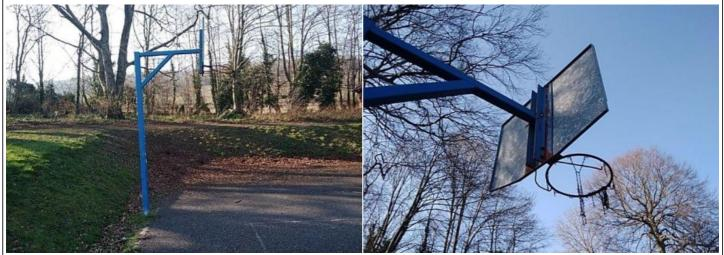
**Finding:** The paintwork on this item has been damaged or worn exposing the metal underneath which is rusting
