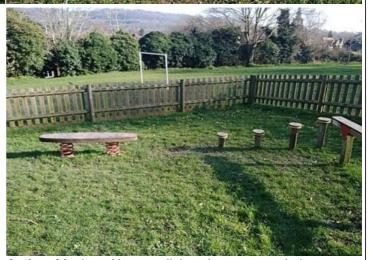
**Finding:** The step between the items is quite large and users may not be able to complete the step without touching ground, the items could therefore be considered to be within the falling space of each other, however the intention of the play activity continuity is easily apparent and foreseeable to the user
