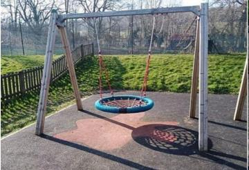
Finding: The seat has been installed incorrectly and needs Action: Reinstall the seat in the correct orientation rotating by 90 degrees to ensure that the eyelets are at the same angle as the suspension; these swing seats have less impact attenuating properties to the sides of the seat than to the leading edges
