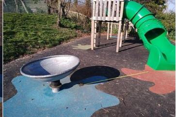
**Finding:** The falling space overlaps the free space between **Action:** Monitor - No remedial work recommended the dish roundabout and the slide in contravention of the requirements of BS EN 1176:2017 Part 1
