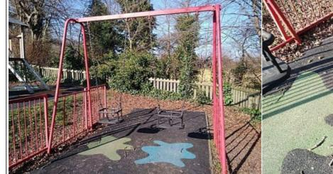
**Finding:** The chain openings are in excess of 8.6mm and do not meet the recommendations of BS EN 1176 Part 1
